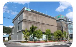
LCV Data Center
