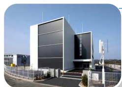
Okayama Data Center
