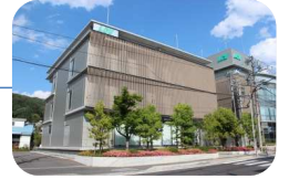
LCV Data Center
