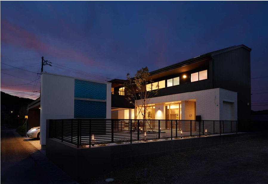
(Pic. 3: OTS House at night. Exterior and passive design achieve both self-sufficiency and aesthetics by enhancing the beauty of nature)
