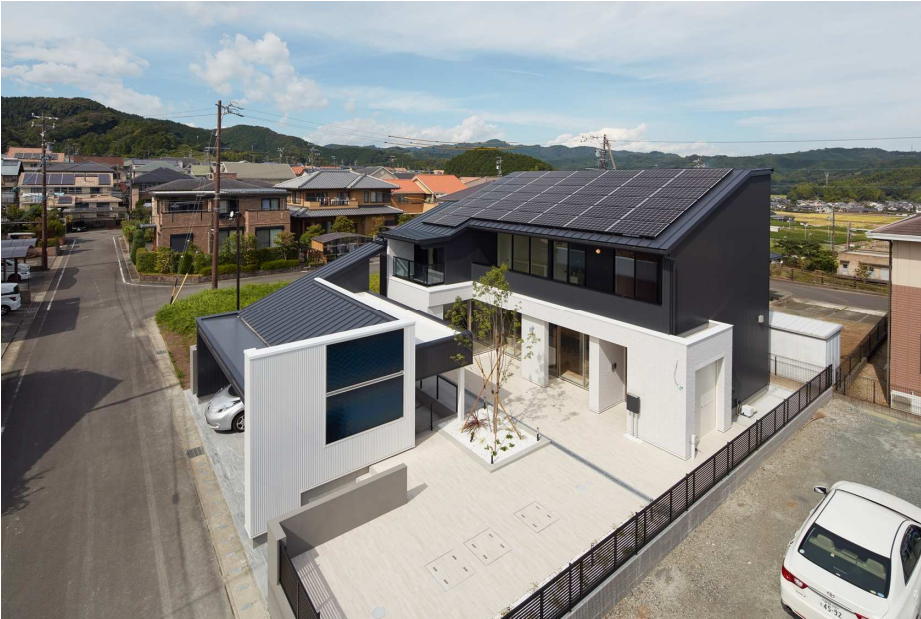
(Pic. 1: Full view of OTS House taken by the drone. The roof sloped to one side and the vast inner court to collect rainwater efficiently. A rainwater tank is buried under the court, which can store a maximum of 10,000 liters of water.
